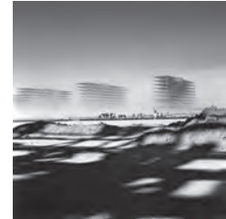
Fig. 2 Marcel Gautherot The Ministerial Edifice under construction , c. 1958 Épreuve gélatino-argentique Instituto Moreira Salles © Marcel Gautherot / Instituto Moreira Salles
