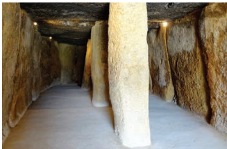
Monolithic pillars dividing a large chamber into two aisles, Menga, Spain, 4 th millennium BC / Photo Olaf Tausch.
