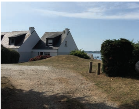
Etal-Berder tumulus in the middle of a private housing development, Larmor-Baden, Brittany, France.
